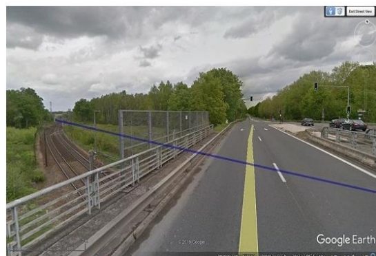
Figure 3f: Same Bridge in Street View (in Google Earth)
