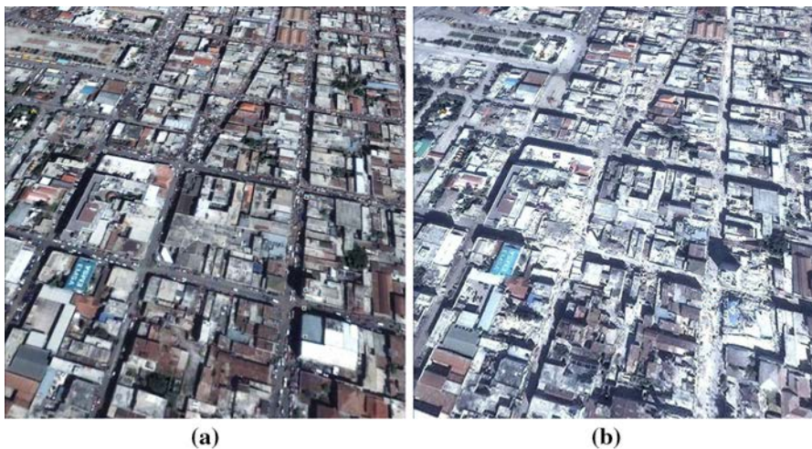
Fig. 1 One sector of Port-au-Prince 1 day before (a) and after (b) the 2010 earthquake (Source: Google Earth 2016)
